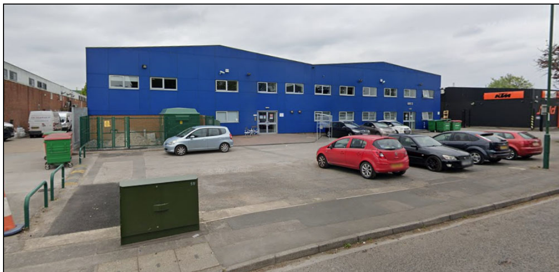
Figure 2: View of Site from Little Tennis Street
