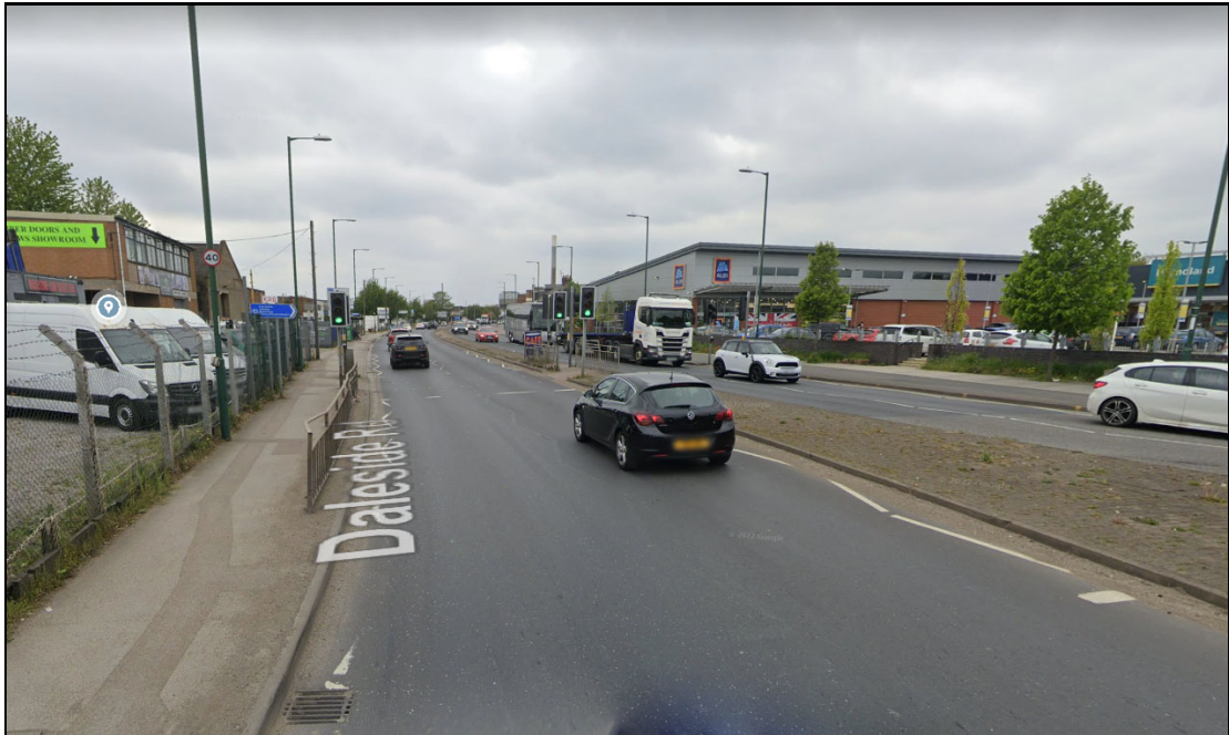
Figure 6: Footways and Pedestrian Crossing on Daleside Road
