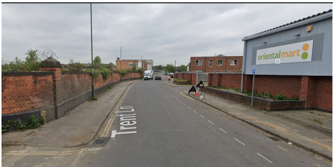
Figure 5: Footways on Trent Lane
